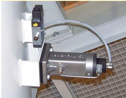
Filter outlets cleaning
